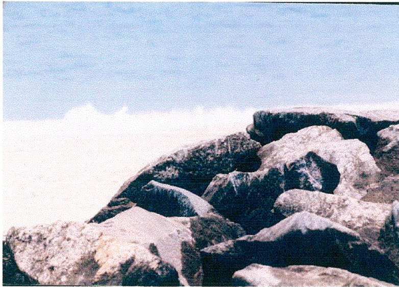
Sea Wall is made up of boulders
